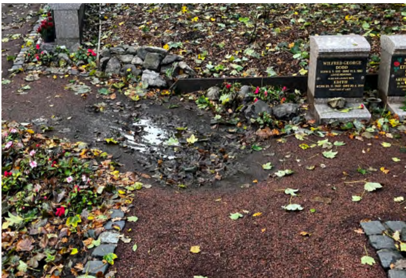
Failing old sections of pedestrian paths need to be repaired to avoid claims so rationalisation of path surfacing and hardstanding will reduce this ongoing burden.
