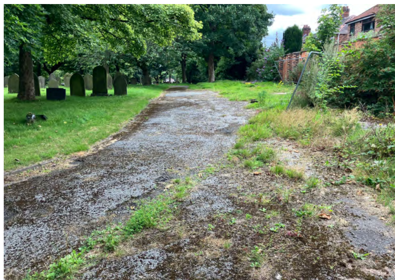
Excessive areas of redundant hard standing proves both expensive to maintain but also an issue in ever increasing heavy rain and cloudbursts with high amounts of surface water run off.
