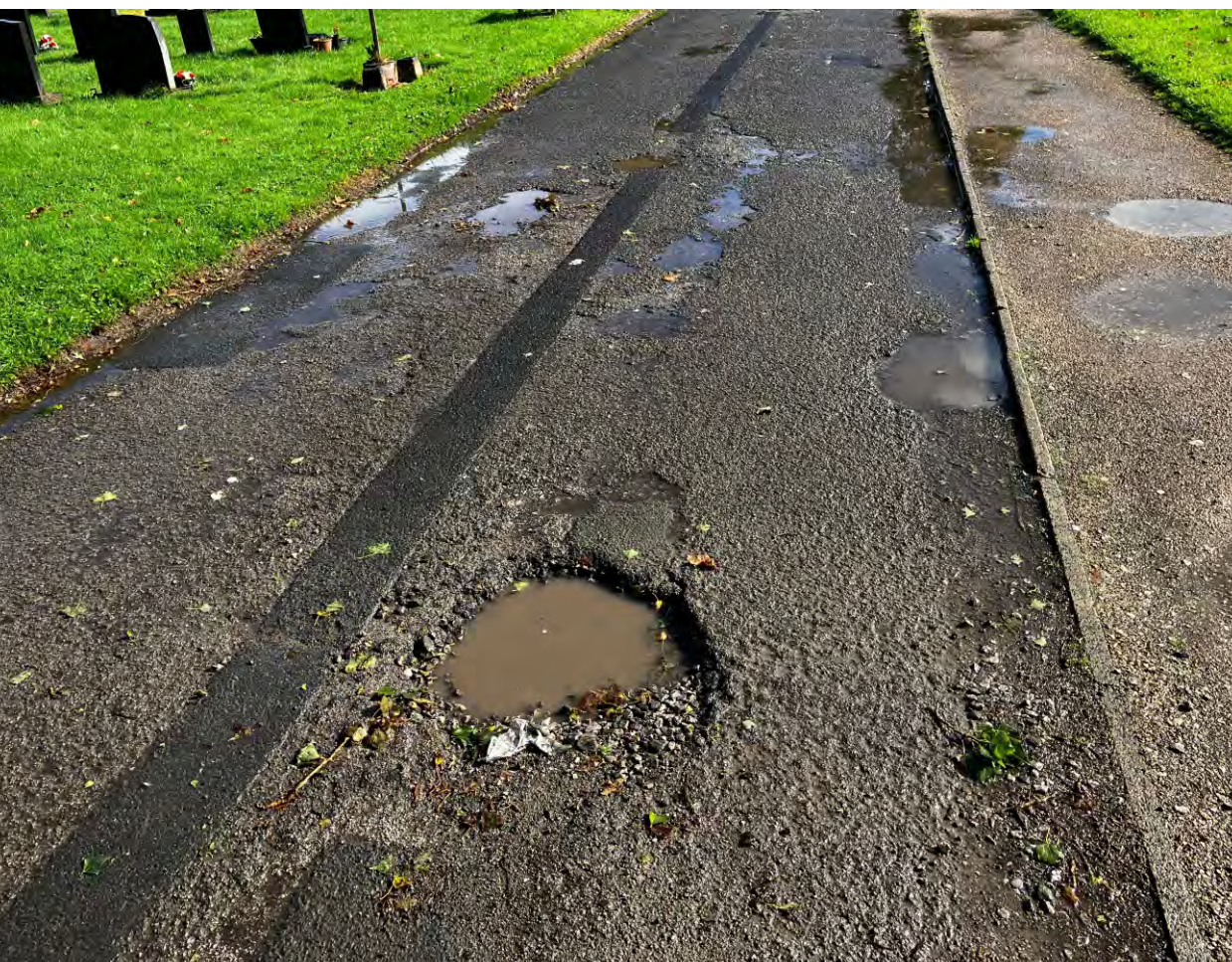
Occurance of potholes is common across wide expanses of bitmac and both proving expensive to repair and deal with resulting claims from trips and damage to vehicles.
