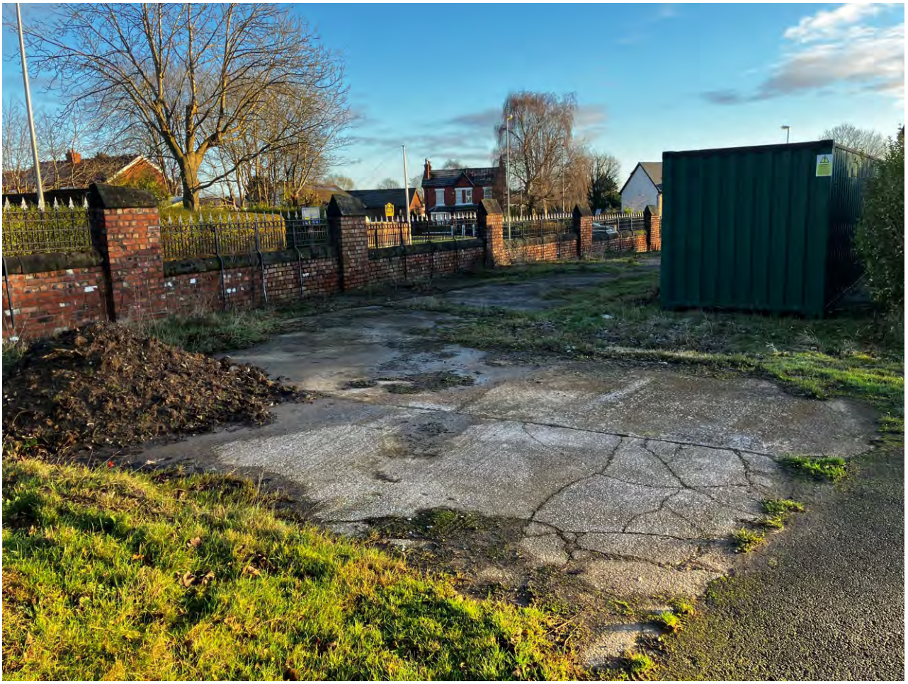
Derelict hard surfacing does not allow filtration and is unsightly so will be removed and replaced with green infrastructure.
