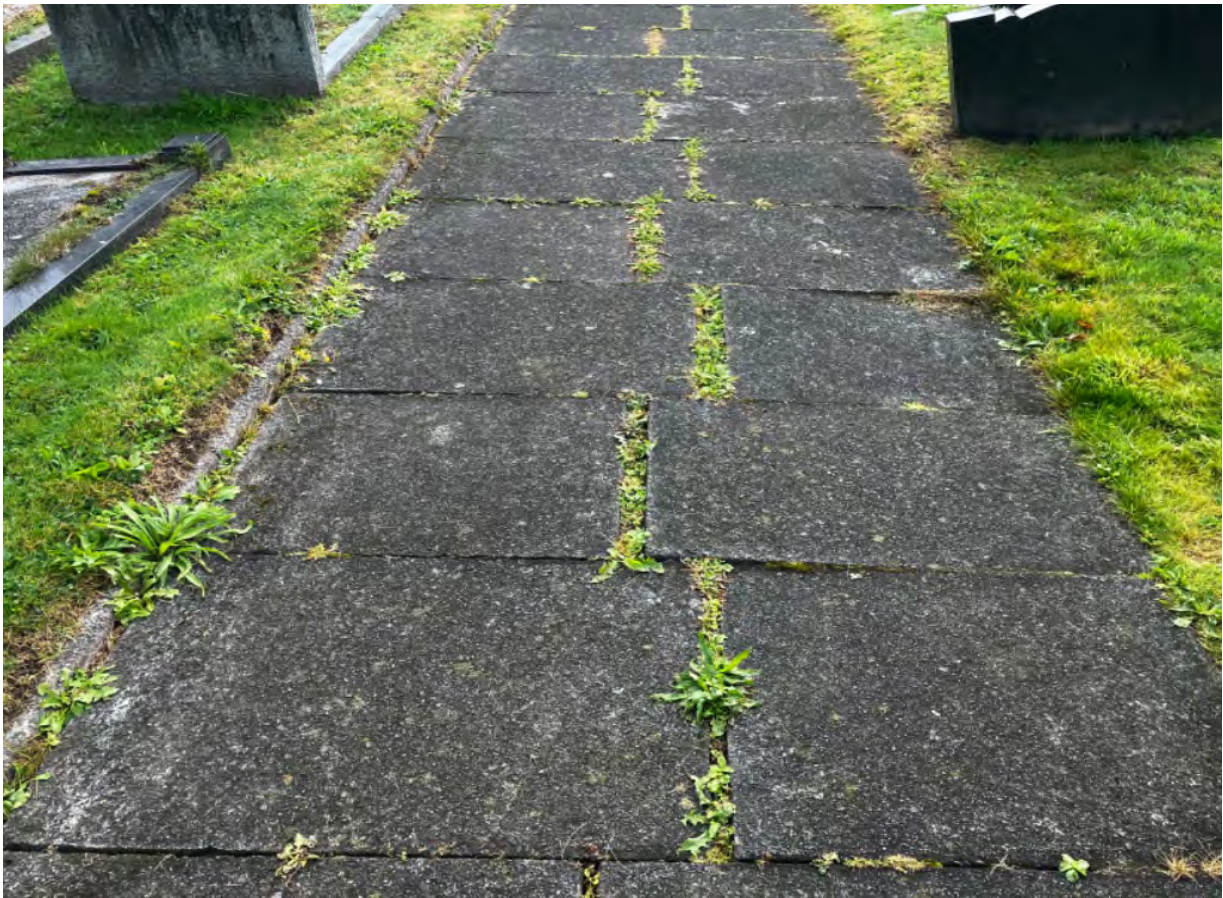
The existing paving slabs forming pedestrian paths are uneven and have become a trip liability, providing an ongoing maintenance issue.
