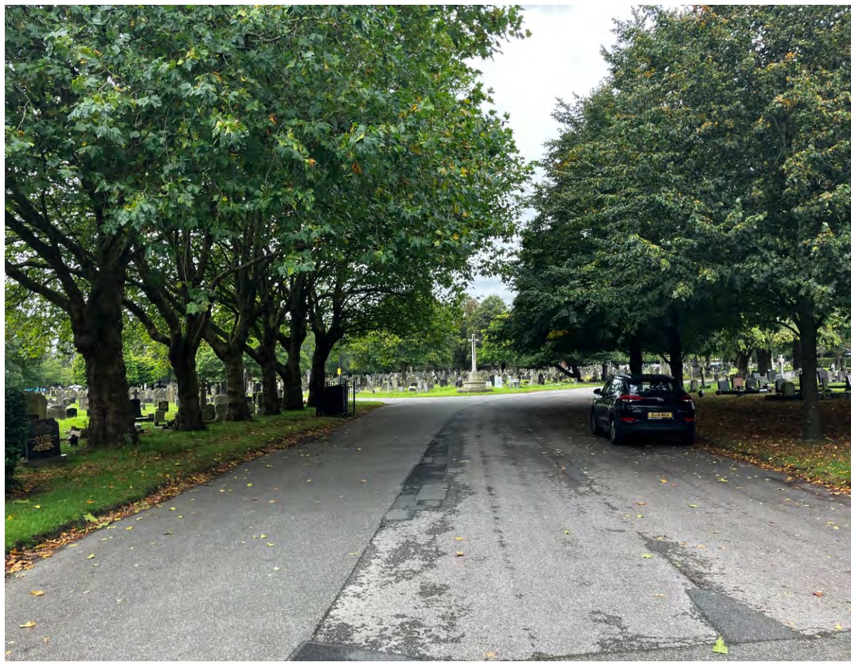
Excessive carriageway width with large expanses of bitmac surfacing has proved both expensive to maintain but also an issue in ever increasing heavy rain and cloudbursts with high amounts of surface water run off.
