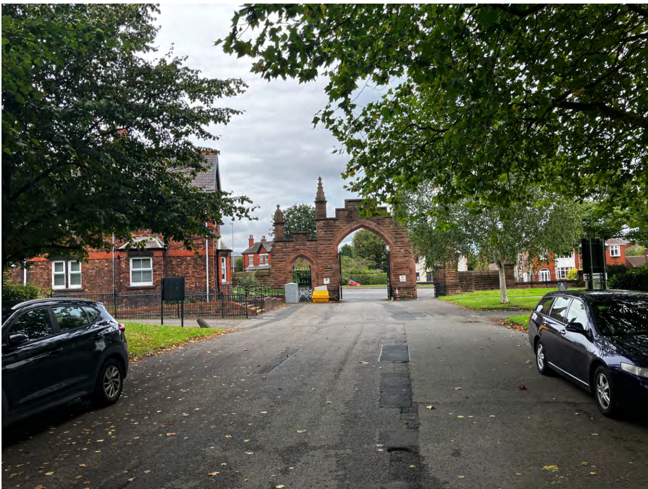
Excessive carriageway width with large expanses of bitmac surfacing has proved both expensive to maintain but also an issue in ever increasing heavy rain and cloudbursts with high amounts of surface water run off.
