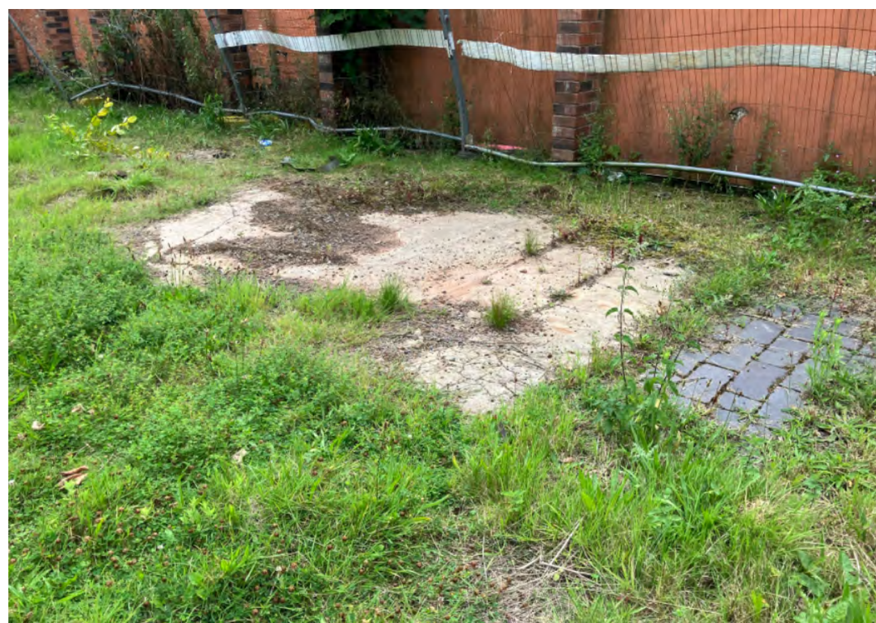
Excessive areas of redundant hard standing proves both expensive to maintain but also an issue in ever increasing heavy rain and cloudbursts with high amounts of surface water run off.
