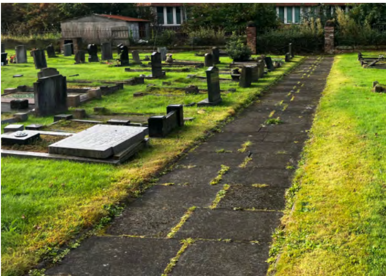
The existing paving slabs forming pedestrian paths are uneven and have become a trip liability, providing an ongoing maintenance issue.
