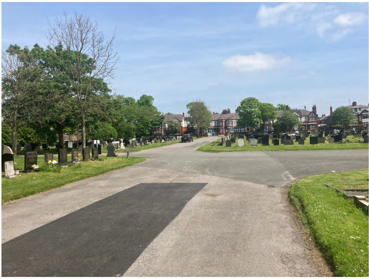
Excessive carriageway width with large expanses of bitmac surfacing has proved both expensive to maintain but also an issue in ever increasing heavy rain and cloudbursts with high amounts of surface water run off.
