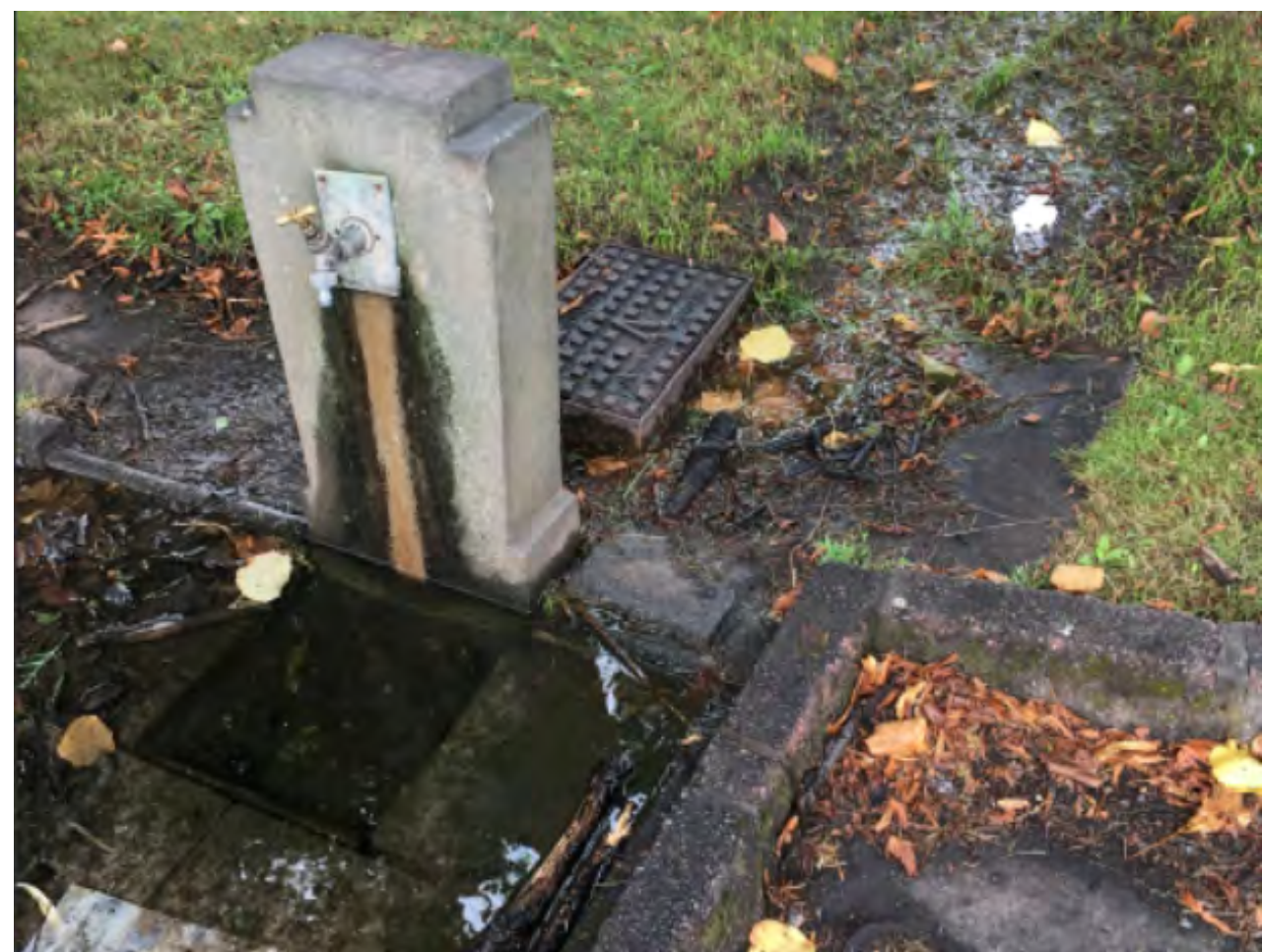
Old failing watering points are becoming a problem with expensive leaks and need to be replaced.
