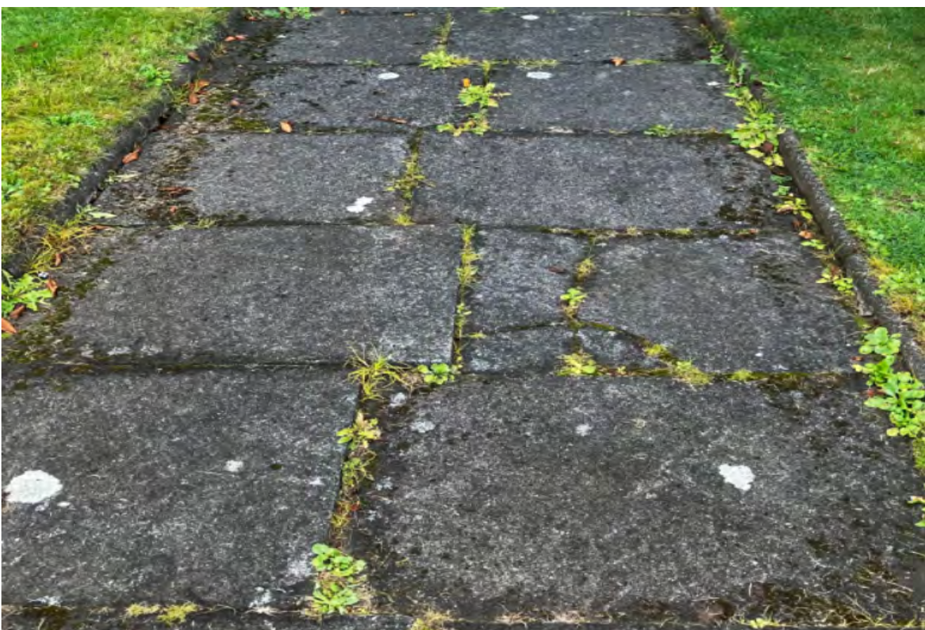
The existing paving slabs forming pedestrian paths are uneven and have become a trip liability, providing an ongoing maintenance issue.
