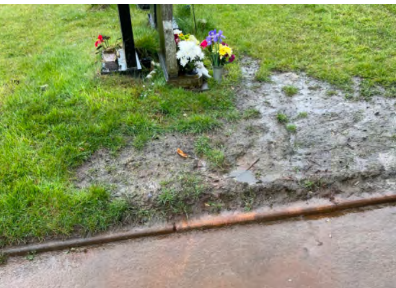
Flooding during heavy rain and cloudbursts is an ongoing issues in the cemetery around some grave plots and requires solutions to slow or direct surface water run off.
